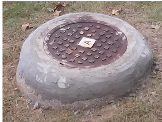
After--Note how the lip has been repaired
